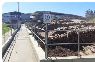
The sawmill produces 90% of CHEP SSA's annual pallet purchases, and 40% of the repair material, with timber supplied to exact CHEP dimensions, maximising timber yield.
