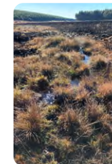
CHEP is undertaking remediation works to protect waterways and enhance ecological function.
